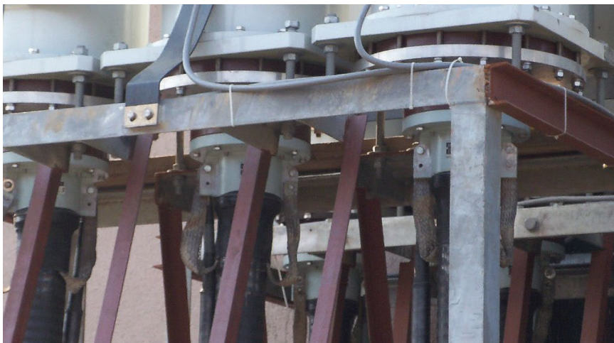
PATR140-SF terminations installed in a GIS.
