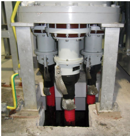
SSC140-SF terminations installed in a GIS.
