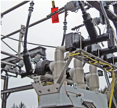
Figure 11: Elbow-Connected G&W Viper Reclosers
