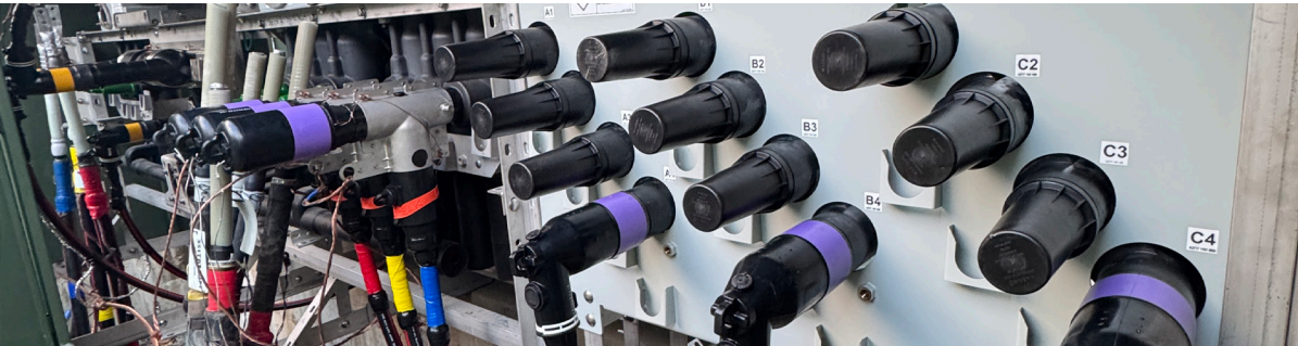
G&W Electric padmount solution with multi-way Trident® solid dielectric switchgear (shown on left) and 4-position junction bar (shown on right) in common enclosure application.
