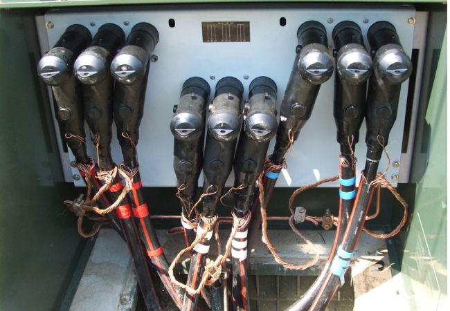
Cabinet with three 3-position junction bars
