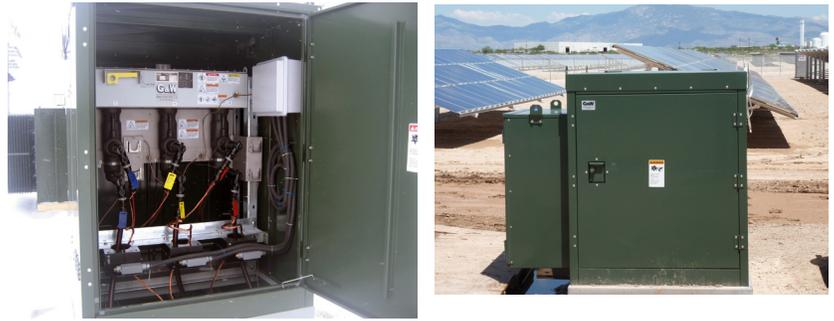
Padmounted Viper-S used in place of a circuit breaker in a solar generation intertie application
