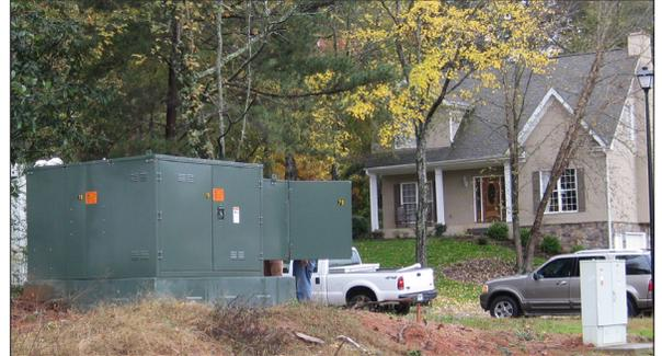
Image 1: Padmount switch with side control enclosure.
