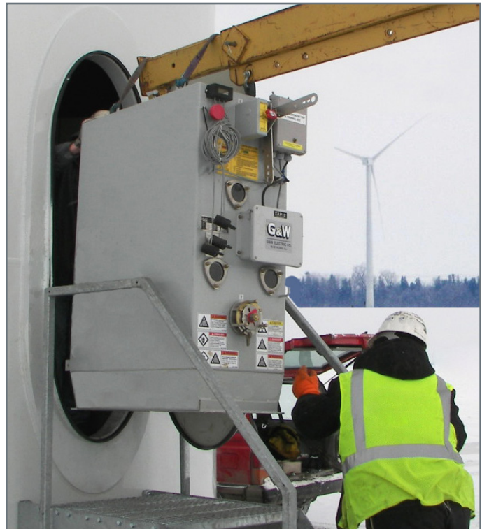
▲ Compact vertical design fits through the typical entrance opening for installation after the tower is constructed.
