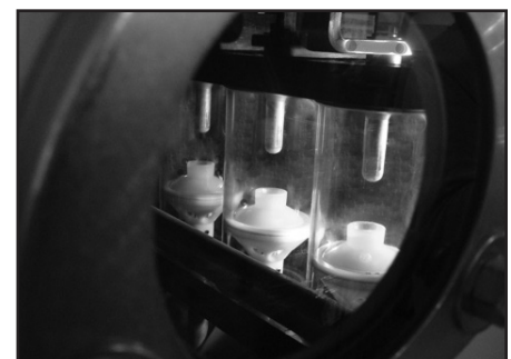
▲ Load break switch visible break.
