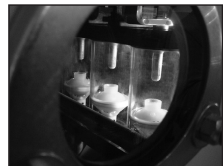
▲ Load break switch visible break.
