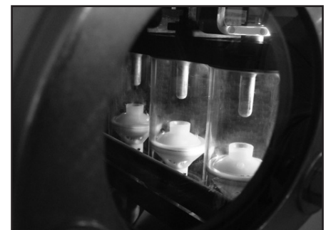
▲ Load break switch visible break.
