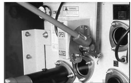
▲ Load break operating handle.
