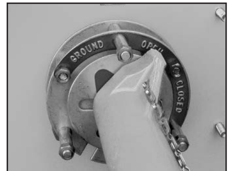
▲ Load break multi-position switch operator.
