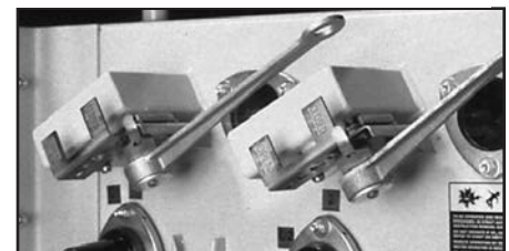
▲ Hookstick operable load break handle.
