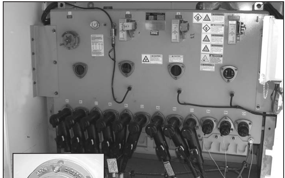
▲ Front access PNI with load break rotary operator and interrupter single operating handle.
