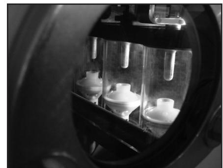
▲ Load break switch visible break.
