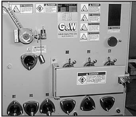
▲ Canister fuses incorporate a provision for hookstick removal and replacement.
