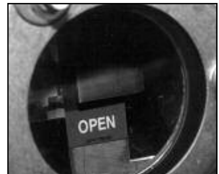
▲ Fault interrupter position indicator.
