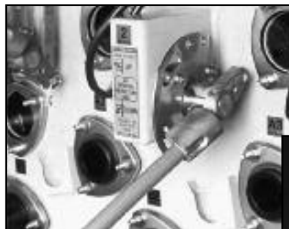
◀ Three phase interrupter operating handle for manual three phase operation and reset.
