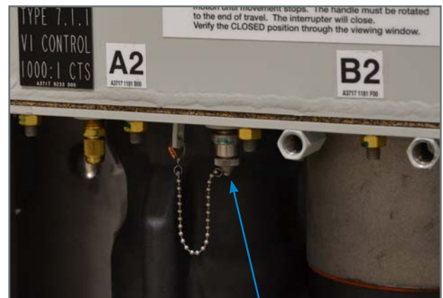
▲ Type 7 control programming port
