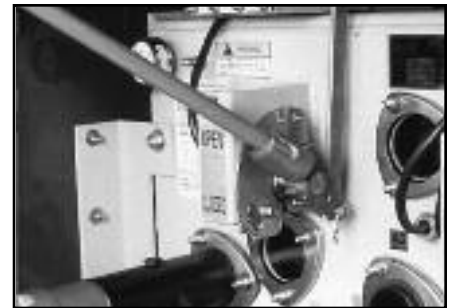
▲ Load break operating handle.
