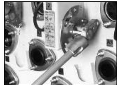
▲ Fault interrupter operating handle.
