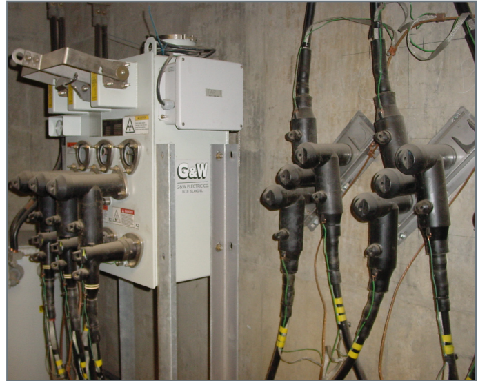
▲ Vacuum interrupter switch provides overcurrent protection while the 600A junctions provide a disconnect point.
