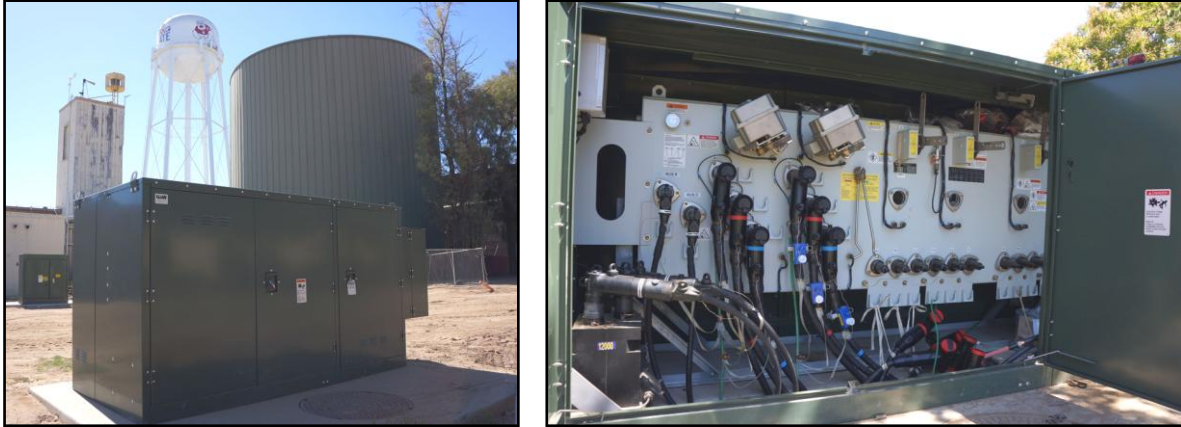
Figure 7: SF6 insulated 6-way padmount switch
