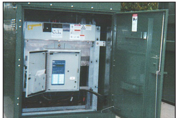
Recloser front view with SEL 351-R control
