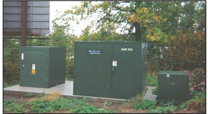
Padmount recloser (left), three phase stepdown transformer (center) and single phase transformer.
