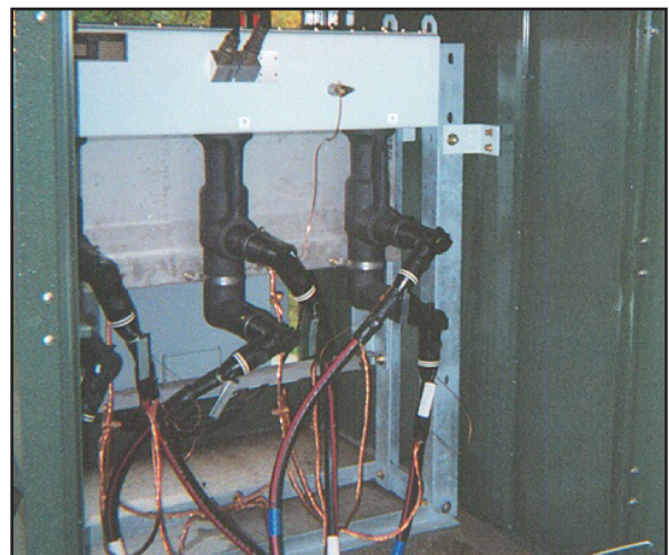
Recloser rear view cable connections
