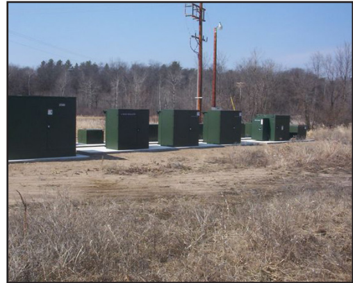
15kV Viper-S Z module recloser with SEL 351-R control.
