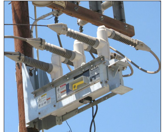
Image 2: G&W 38kV Viper-S recloser with "Z" modules.
