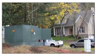
Image 1: Padmount switch with side control enclosure.
