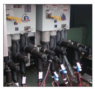
Image 2: Front/back access padmount switches incorporated two Trident-SR switches on both sides.
