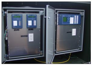
Image 3: SEL-751As and 451 were mounted in a common enclosure on the side of each switch.
