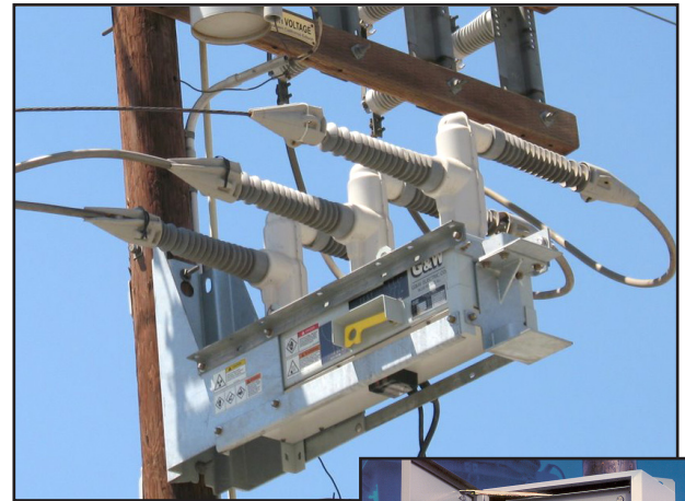
15kV Viper-S Z module recloser with SEL 351-R control.
