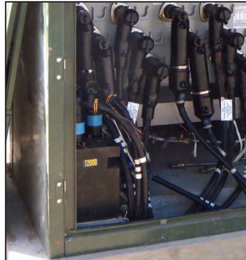
▲ External CPT installation
