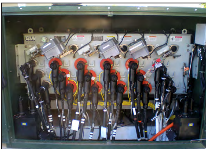
▲ Automated switch retrofit installation.
