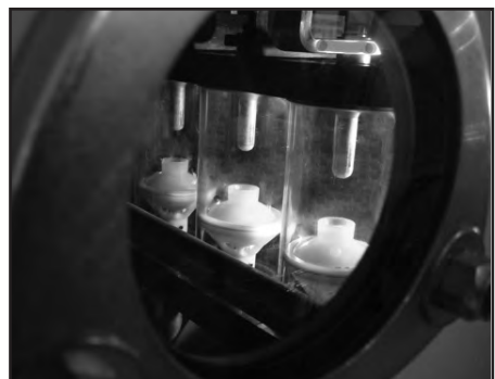
▲ Load break switch visible break.
