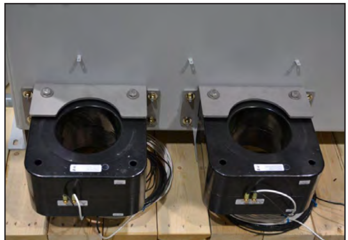
▲ External CT Installation
