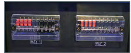
▲ ABB FT1 test switches
