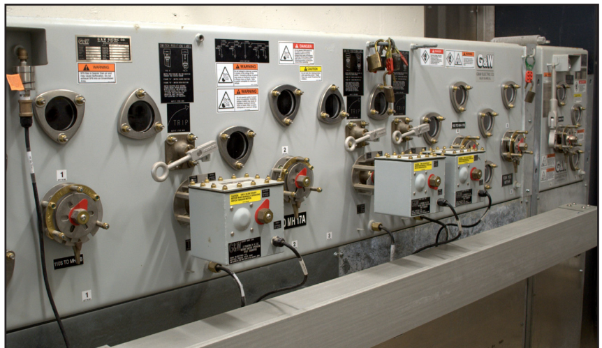
▲ SF6 Bus Tie Switch
