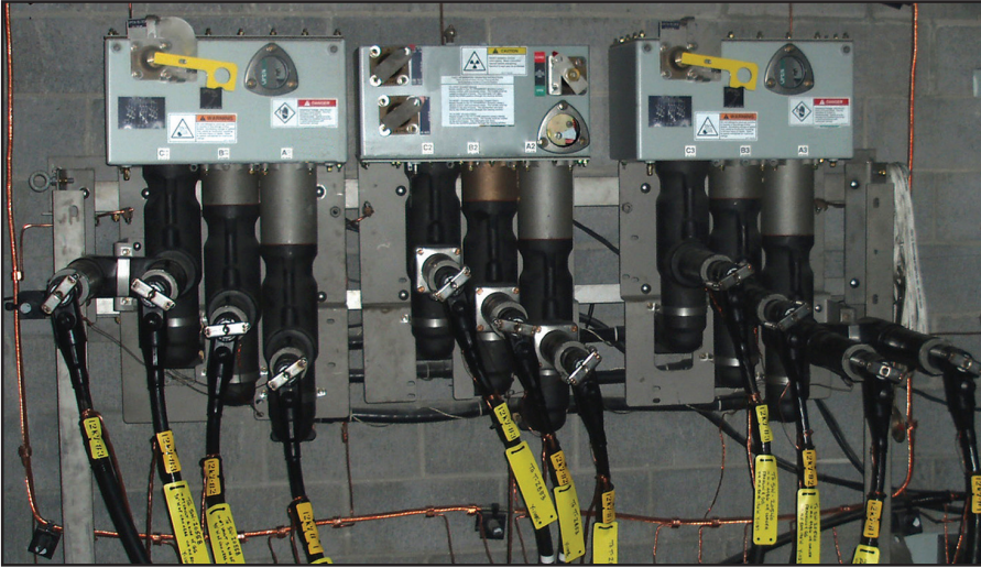
▲ Magnetic Actuated Trident-SR multi-way in a submersible vault installation.
