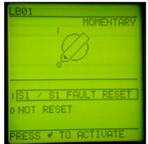
▲ Faulted circuit indicator reset
